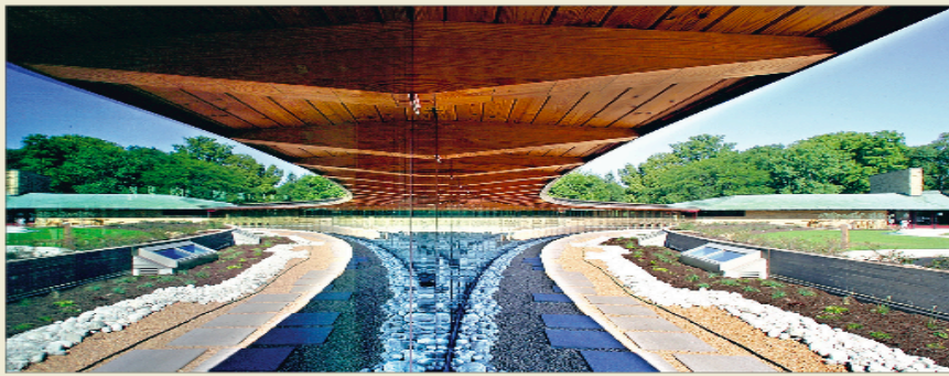
The view from the windows of the semicircular addition to the First Unitarian Church provides a mirror image of the addition and its connection to the original Frank Lloyd Wright-designed church. Architects chose a gentle curve to contrast with the sharp angles Wright chose.
