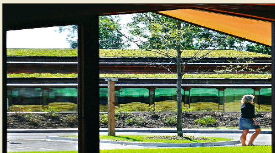
ABOVE: Among the green features of the addition is a roof planted in sedum, which will need to be weeded but not mowed. The roof helps control runoff and keeps the building cool in the summer.
